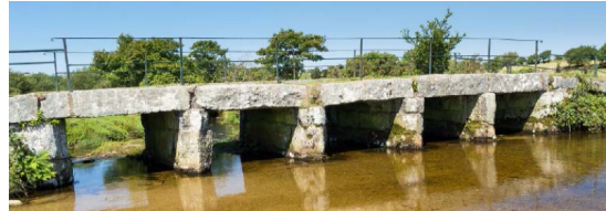
Simple bridge design with beams and pillars
