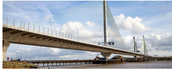
Mersey Gateway Bridge, designed by Knights Architects and opened in October 2017.
